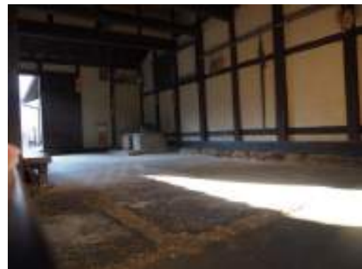
Fig.5.5 Machiya Shiryōkan, Uchiko, 2015. The front and the courtyard are connected by a tōridoma rebuilt as its original state.
