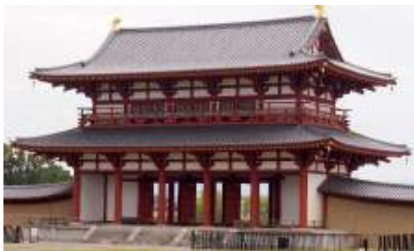
Fig.2.8 Suzakumon, Heijōkyō, Nara, 2015. The reconstruction of the gate was finished in 1998, after an archaeological study to bring the remains of the foundations up, and a re-design based on different sets of fukugenzu drawings. The drawings were based on analogies of structures in and around the old capital.
