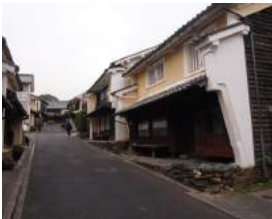
Fig.3.4 Sodekabe, lateral wall standing out of the façade of a machiya , Uchiko, 2015.
