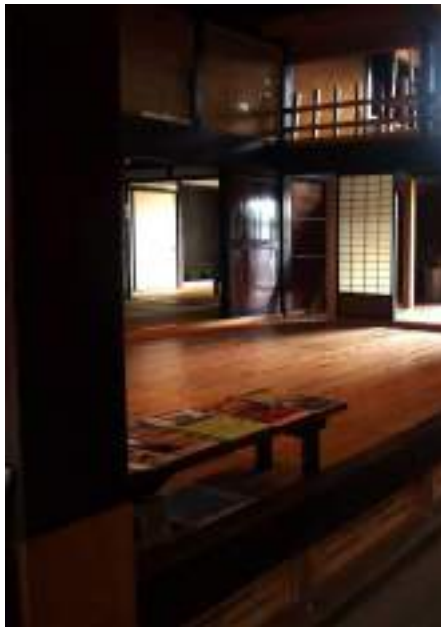
Fig.4.51 Kyūmakitake house, Kurayoshi, 2016. Intervention with old and new elements in different colours, being newly introduced elements in a lighter colour so that they can be distinguishable.
