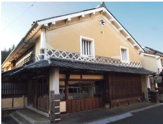
Fig.4.45 Façade restored in Yōkaichi Gokoku district, 2015. The lattice in the first floor was newly introduced. It was incompatible with the pre-existent structure, with decorative corbels under the rood structure. The pillar at the left has its corbel, while the rest had to be removed to build the lattice.
