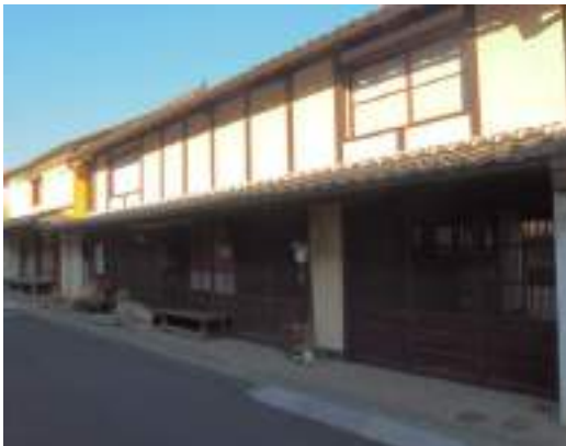
Fig.3.15 House with shinkabe Wall (the structure is visible), 2015.
