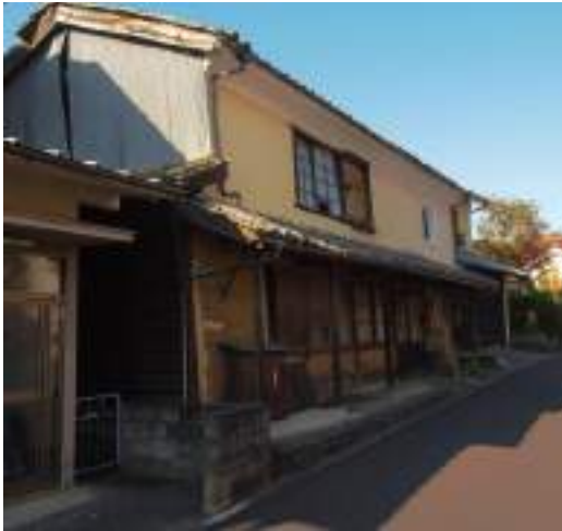
Fig.3.14 House with ōkabe Wall (the structure is concealed inside the wall), 2015.
