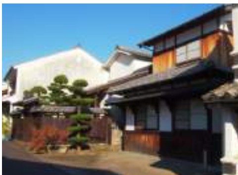
Fig.3.23 Yōkaichi district, 2015. According to Machinami Hozon Center, works in this house conducted before the denken chiku designation turned the roof structure 90 degrees, so that the eaves would be facing the street, as in the traditional houses of Uchiko.
