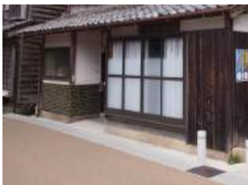
Fig.4.49 Ine, 2016. The privacy given by lattices is obtained with translucent glass.
