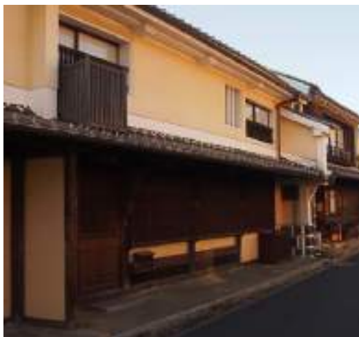
Fig.3.20 Building with a T-shaped sodekabe, 2015. The namakokabe square-pattern is also at the base of the sodekabe, to protect it from rain.
