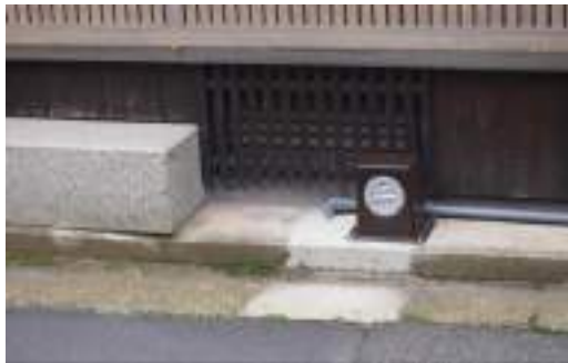
Fig.4.47 Ine, 2016. Ventilation of the sewage system installed by the local government in all the district.
