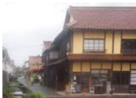
Fig.3.50 Kurayoshi, 2015. Roof with red sengawara tiles. These tiles replaced thatched roofs in the end of 19 th century, to prevent collapses due to frequent snowfalls.
