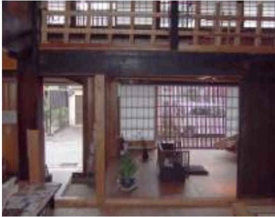
Fig.2.1. Example of material recycling and continuity in Japanese preservation. Kyūmakitake house, Kurayoshi, Tottori. The old pillars have been either maintained or replaced by distinguishable pieces, depending on its state in the present time.
