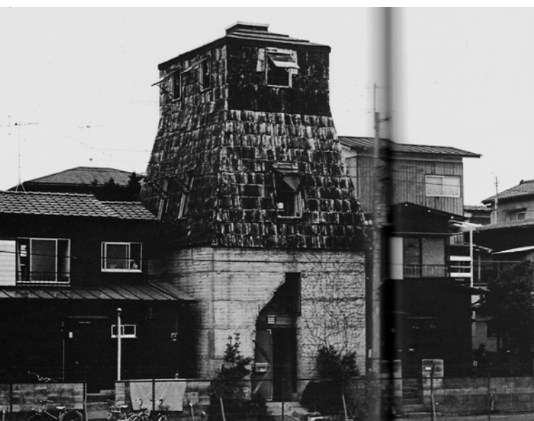
Karasu Castle/ Eiji Yamane / 1970-1972 / Concrete formwork made from steel drums and logs cut and adjusted on site from raw timbe [1]
